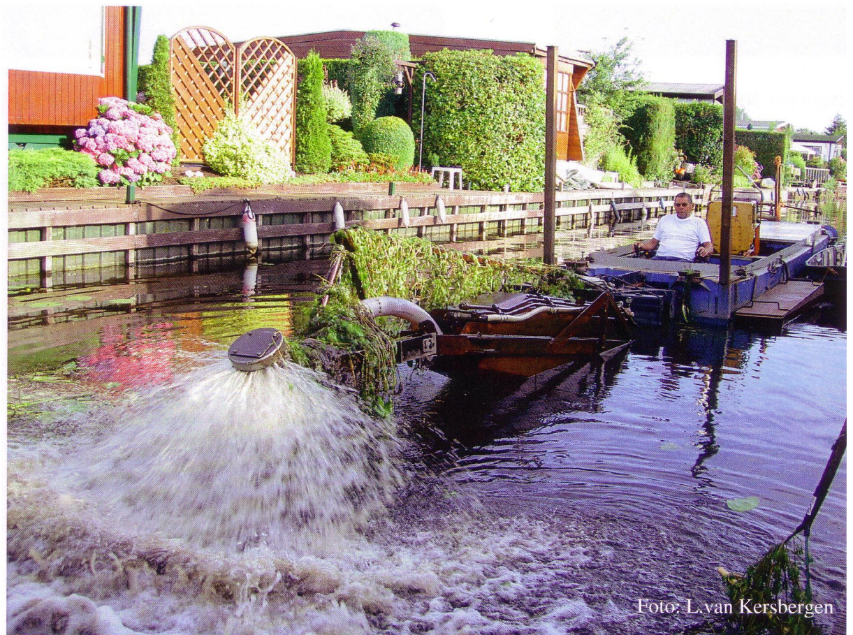
Figure 10. Dredging by the new technique. The head with the water jet is raised above water to illustrate its operation.
